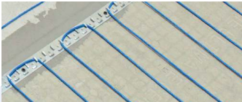
WarmWire installed using CableStrap
